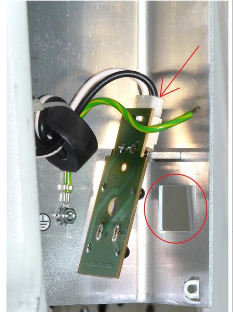
Inside view of obsolete AC power input for BX51. (The AC input receptacle which would be mounted in the empty circled hole had been removed before we received the microscope) Remove AC power lead connection by disconnecting the socket indicated by the arrow above.
