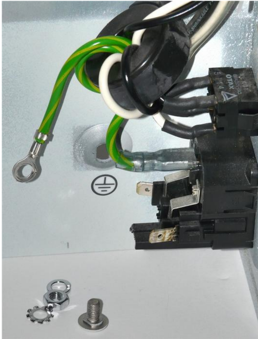
(1) Remove the ground stud. It is not needed as the AC power has been disconnected.
